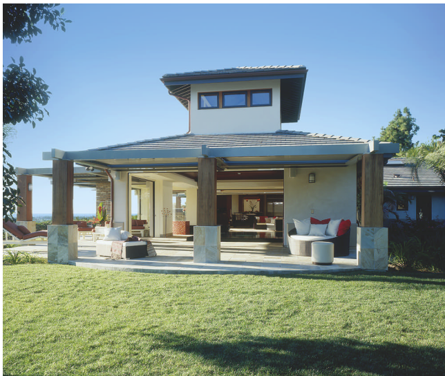
The cupola and clerestory windows above the pool pavilion function as a thermal chimney to release excess heat.
